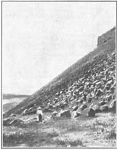
FIG. 21.—The destruction caused by freezing water.
