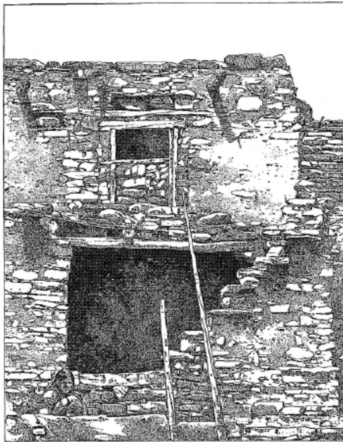
FIG. 79. Rude transoms over Tusayan openings.
