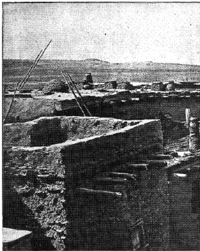
FIG. 34. Stone wedges of Zuñi masonry exposed in rain-washed wall.
