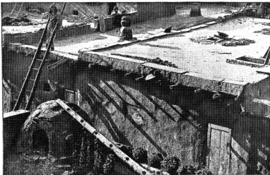
PLATE XCVII. WALL COPING AND OVEN AT ZUÑI.
