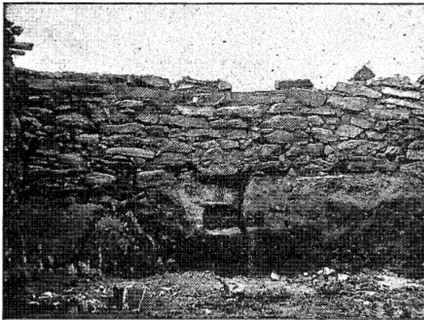
FIG. 35. An unplastered house wall in Ojo Caliente.
