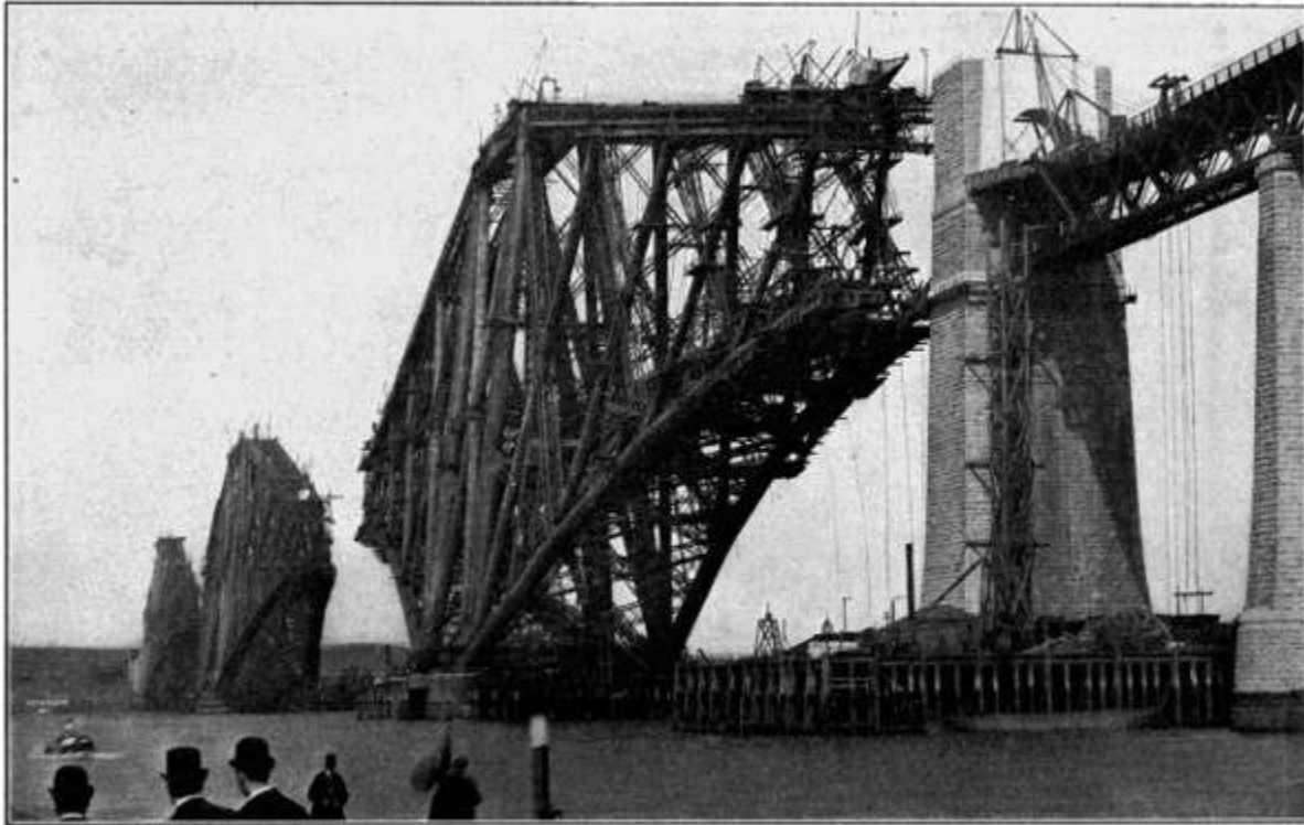
FIG. 228.—THE FORTH BRIDGE. LARGEST VIADUCT IN THE WORLD. FROM A PHOTOGRAPH WHEN IN PROCESS OF CONSTRUCTION. LENGTH, 8,290 FEET; HEIGHT ABOVE WATER, 361 FEET; MAIN SPANS, 1,710 FEET LONG, 150 FEET HIGH.
