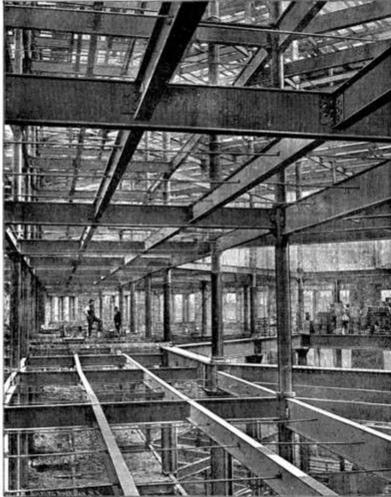
FIG. 235.—INTERIOR CONSTRUCTION MODERN STEEL BUILDING.
