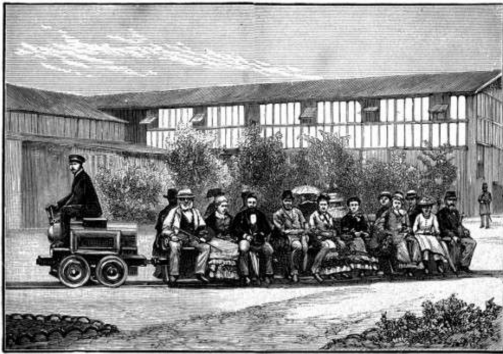
FIG. 33.—SIEMENS' FIRST ELECTRIC RAILWAY.
