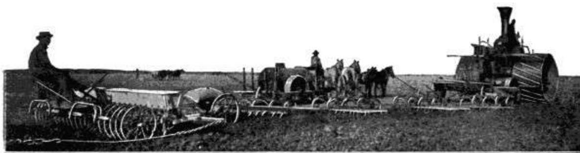
FIG. 158.—FIFTY HORSE POWER STEAM PLANTING COMBINATION.
