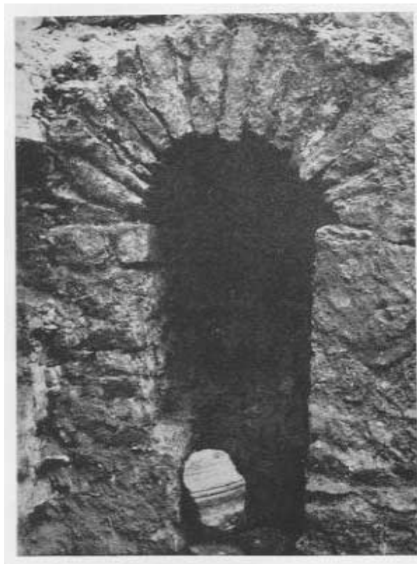
FIG. 28. LINCOLN. SEWER UNDER BAILGATE
