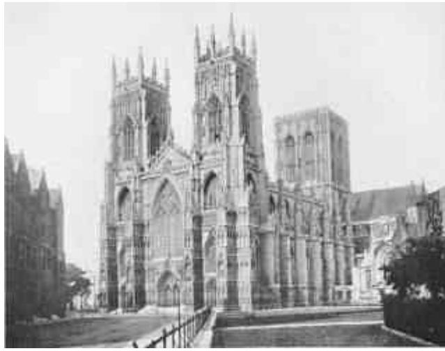
YORK MINSTER. WEST FAÇADE
