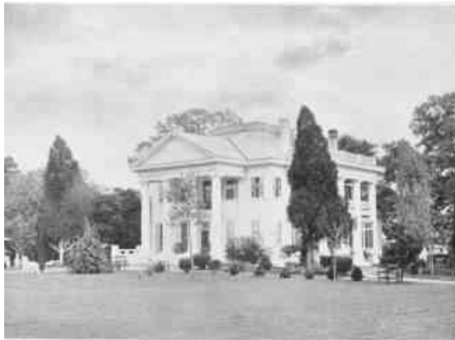
ANOTHER SOUTHERN COLONIAL EXAMPLE, MONTGOMERY, ALABAMA P. 432
