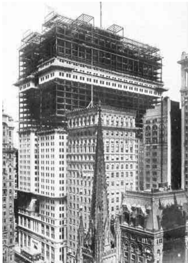
Courtesy of Thompson-Starrett Co. STEEL CAGE CONSTRUCTION
