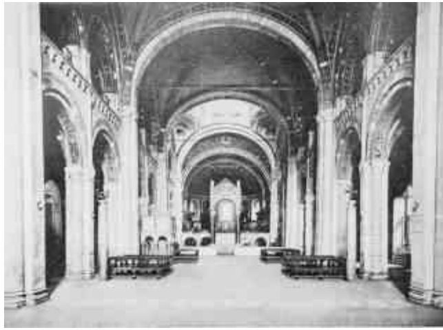
S. AMBROGIO, MILAN EARLY EXAMPLE OF RIB-VAULTING. P.240
