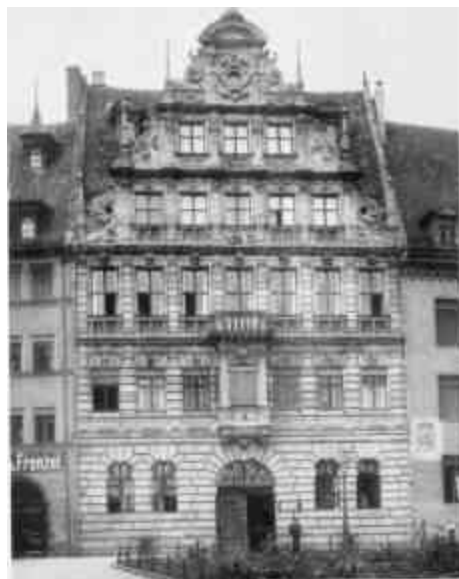
PELLERSHAUS, NÜREMBERG RUSTICATED MASONRY. P. 395
