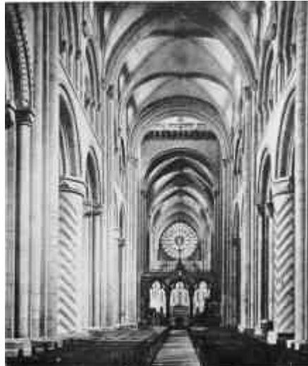
NAVE OF DURHAM CATHEDRAL NOTE THE GIRTH OF PIERS AND CHEVRON ORNAMENT. VAULTING, EARLIEST EXAMPLE IN ENGLAND, COMPLETED 1133. P. 256
