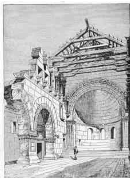
CHURCH OF KALB-LAUZEH, SYRIA SHOWING APSE, WOODEN ROOF, SUPPORTED BY SMALL COLUMNS ON CORBELS; ROUND ARCHES ON PIERS. P. 200
