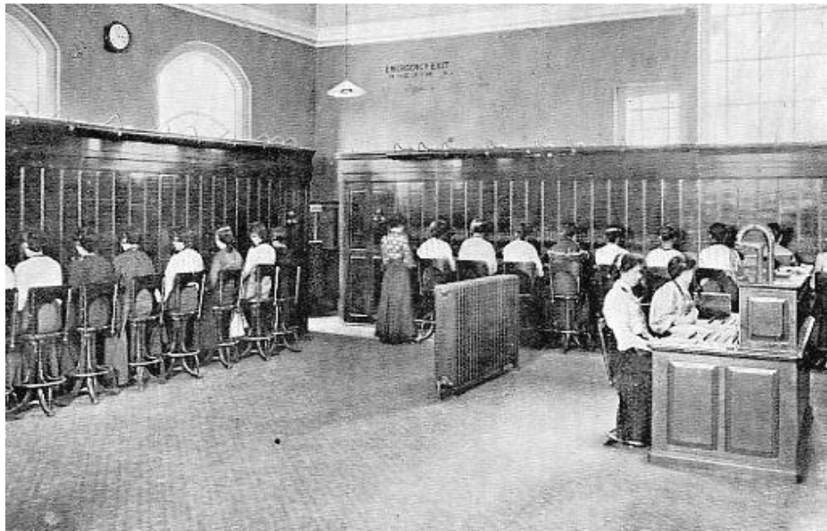
A TELEPHONE EXCHANGE.
