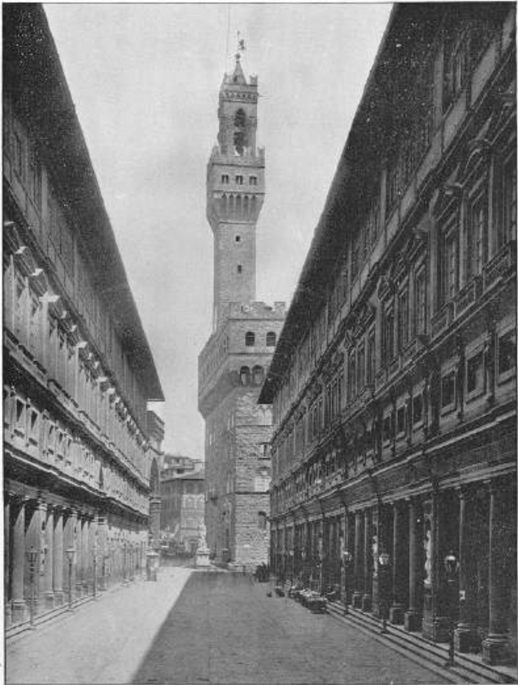
UFFIZI BUILDINGS , FLORENCE, ITALY.—This gallery originated with the Medici collections and was afterwards so improved with the numerous additions by the Lorraine Family, that it is now one of the best in the world, both for value and extent. The Portico of the Uffizi Gallery, seen on both sides of the open court, contains niches, which are adorned with marble statues of celebrated Tuscans. At the farthest end of the court, rises the Vecchio Palace, a castle-like building, with huge projecting battlements, being originally the seat of the Signora, and subsequently used as a casino.
