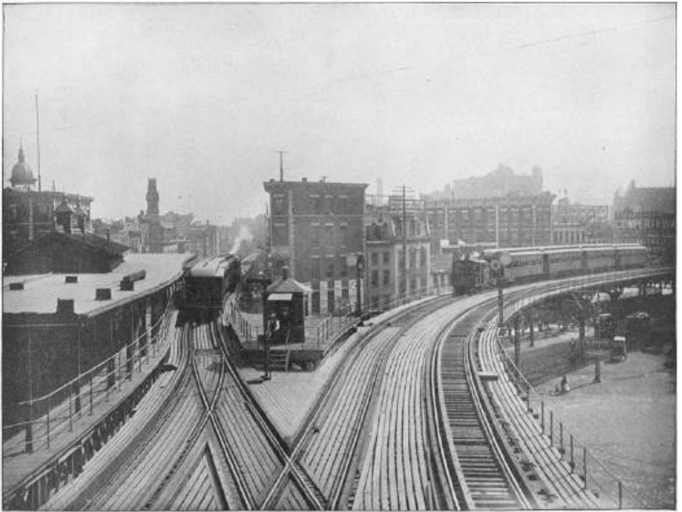
ELEVATED RAILROAD NEW YORK, N. Y.—The steam cars, the street railway and the electric road are the three modern modes of transportation. The motive power of the elevated railroads of New York City is steam, and the quick facilities afforded exceed that of any other country. These elevated railroads are sufficiently high so as not to interfere with street traffic, stations are located every four or five blocks apart, there is little delay, and a passenger can ride from one end of the city to the other in a very short time. It is said that one million people ride daily on the elevated railroads of New York giving the company an income of $50,000 per day. The above photograph represents the railroad at Chatham Square, where it branches off into different directions.
