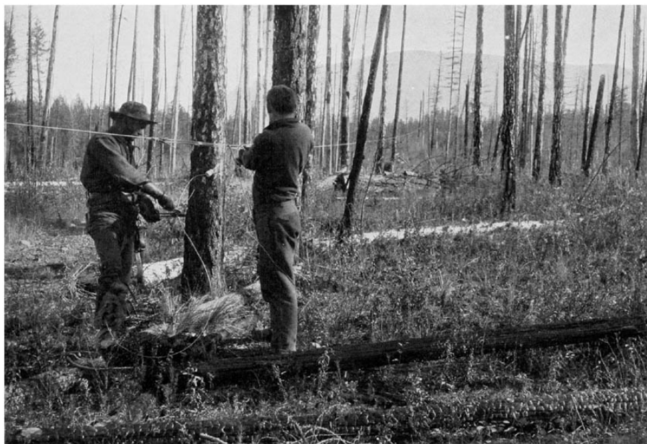
STRINGING A FOREST TELEPHONE LINE
