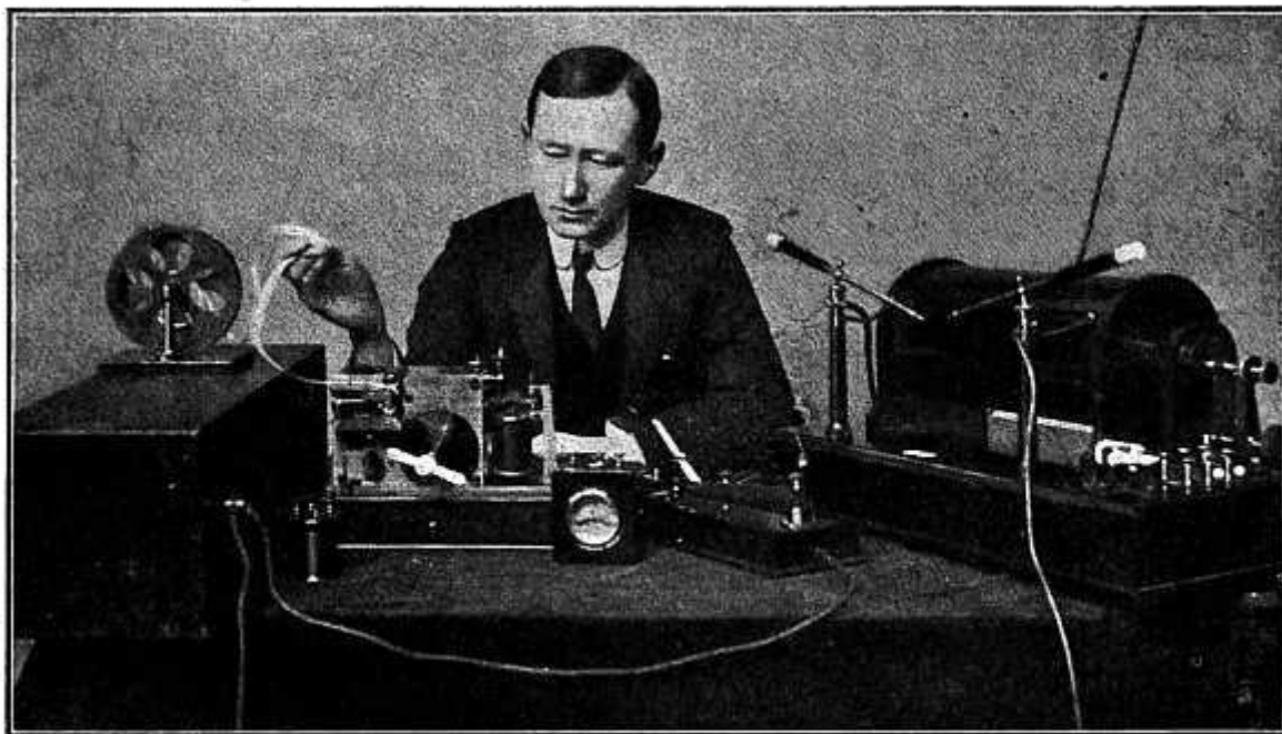
FIG. 108—MARCONI AND HIS WIRELESS-TELEGRAPH SENDING AND RECEIVING INSTRUMENTS
