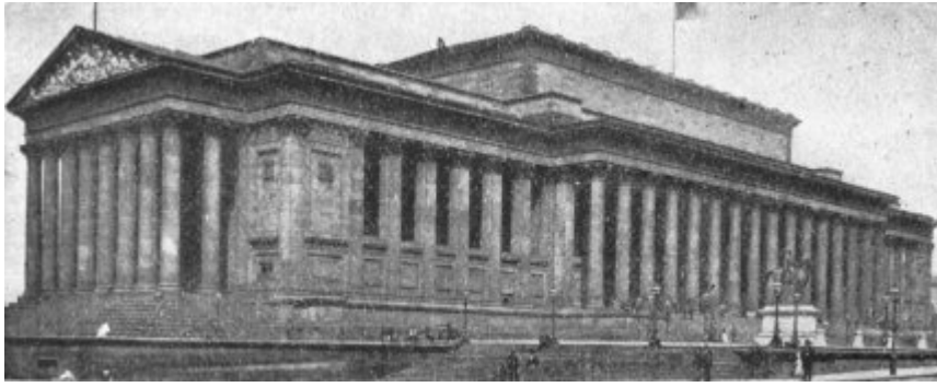
FIG. 199.—ST. GEORGE'S HALL, LIVERPOOL.
