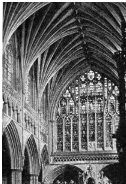
FIG. 129.—RIBBED VAULTING, CHOIR OF EXETER CATHEDRAL.
